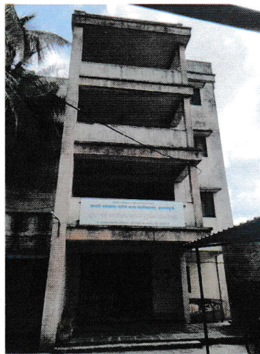
Women's hostel build
